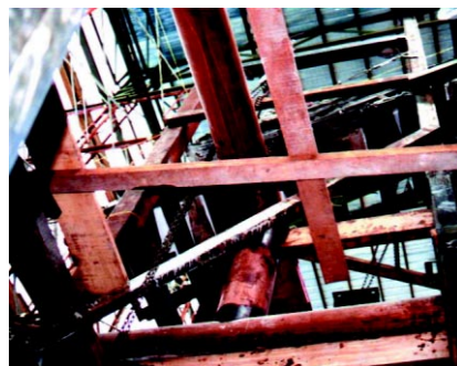
Replacement of Decayed Interactive Structural Members
