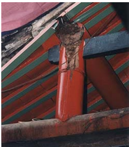
Replacement of Decayed Interactive Structural Members
